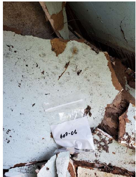
Sample 609-06 Typical Wall Plaster (Debris) Sample
