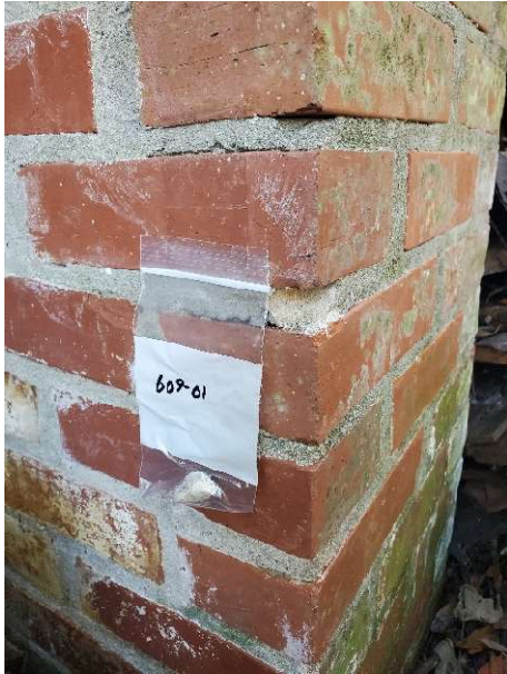
Sample 609-01 Typical Brick Mortar Sample
